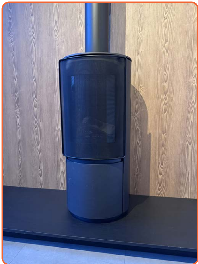
Figure 5.10 | Safety screen installed
